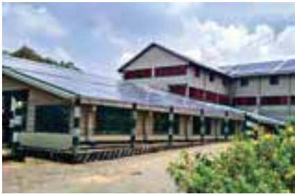
Installed solar panels at Dewalakanda Rubber factory
